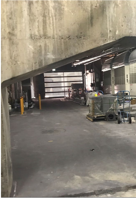
Loading dock viewed from the tunnel
